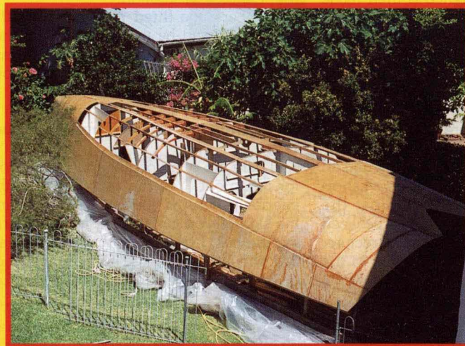
The hull is built upside down. Here, all the longitudinals have been fitted, and the laminated floors and engine bed are also in place.
