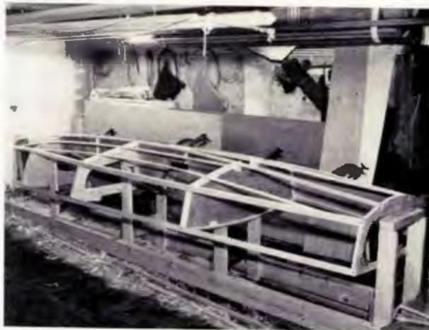
The hull ready for sheathing. There are virtually only three frames, two being watertight bulkheads. Note the change from a V-section at the after end of the platebox to an arc-section at the transom.
