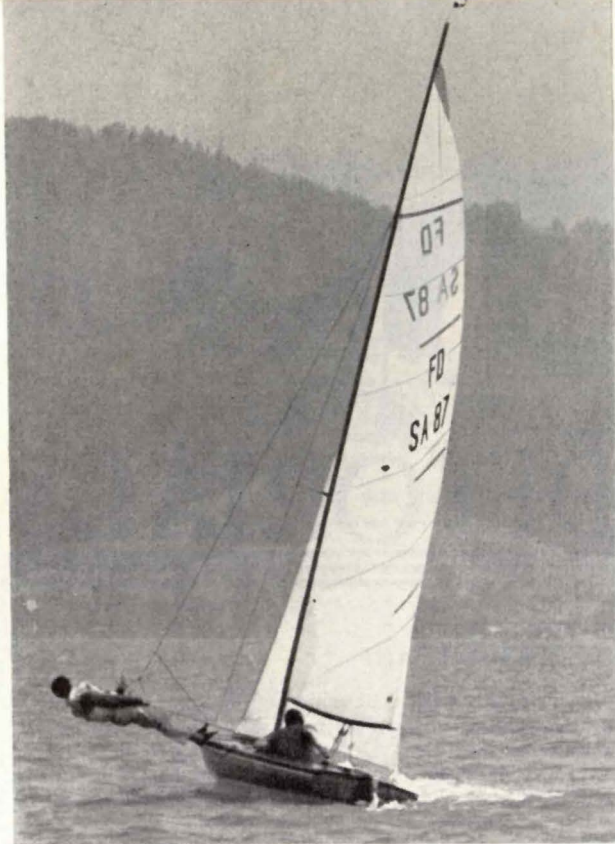
Carmen Stauch hits the most efficient trapeze angle on the Attersee. Note aid given to aerofoil section of mainsail by flexible boom trimming.
